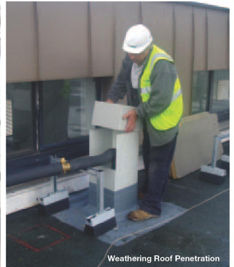
Weathering Roof Penetration
